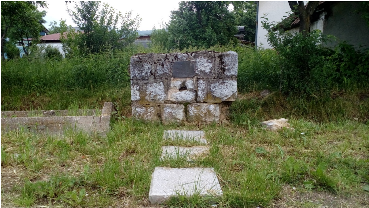
Figure 2a: Fountain in Grlica
