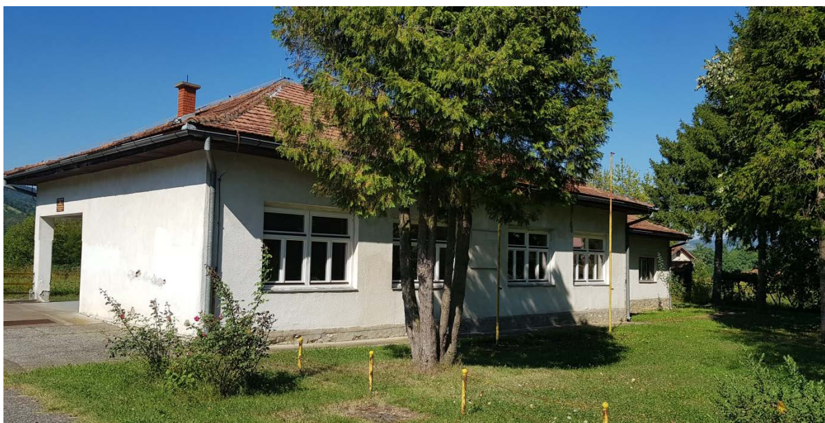
Figure 29a: School building on which the plaque is situated
