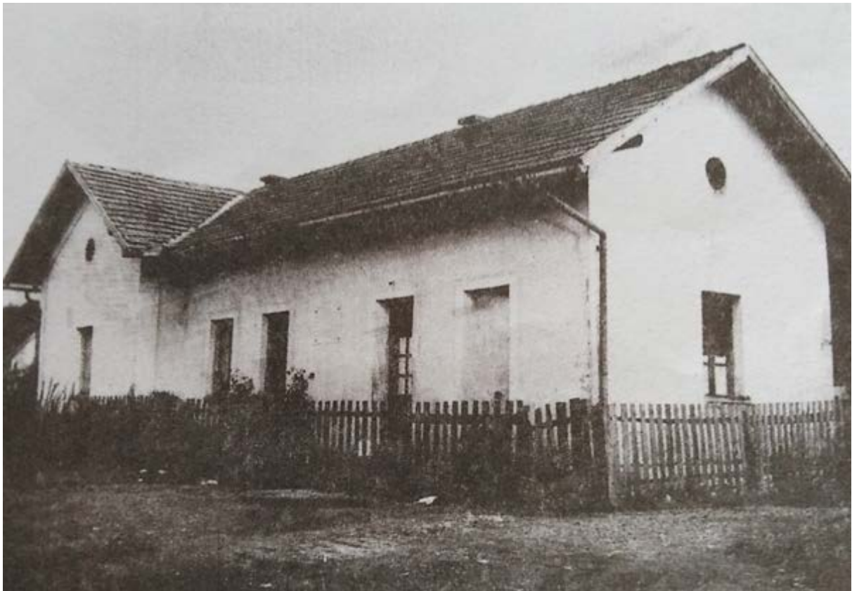
Figure 30a: Train station in the 1980s, with plaque next to door
