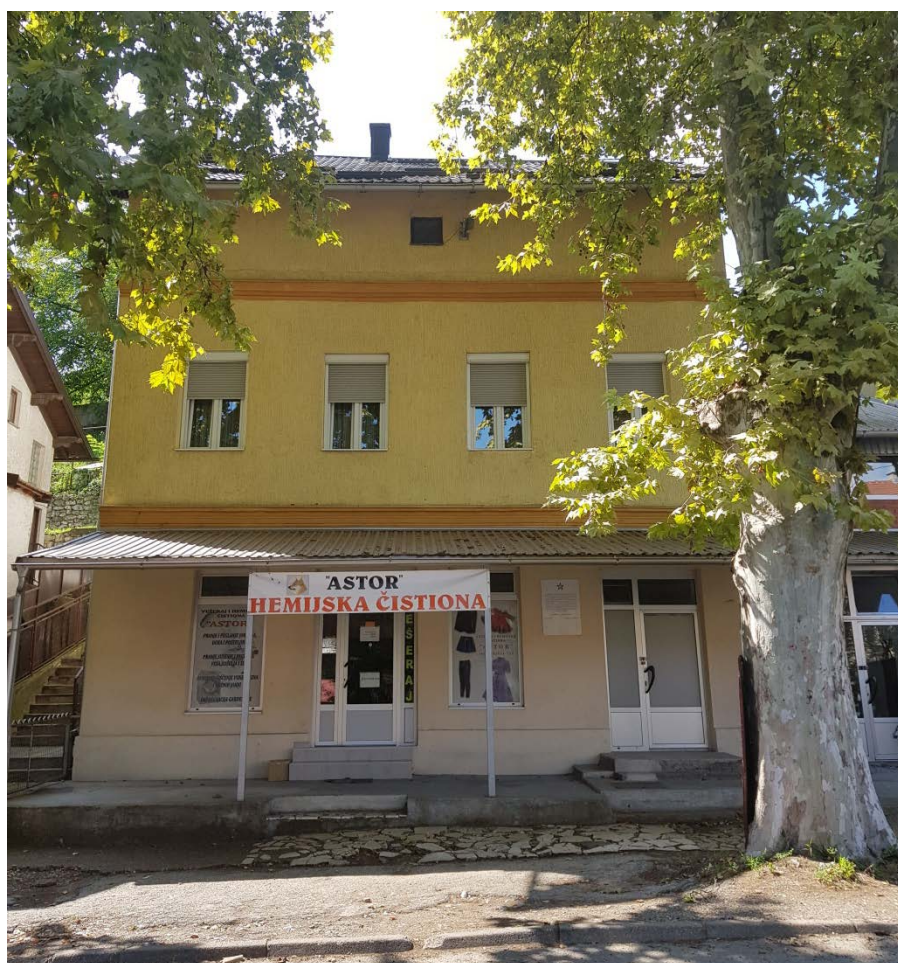
Figure 11b: Present-day appearance of the building, 2019
