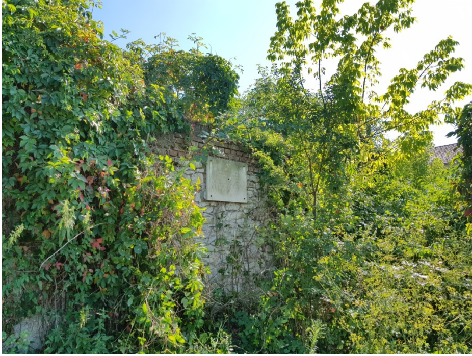
Figure 30c: Plaque after clearance of overgrowth
